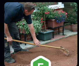
5 Add thin layer of fine aggregate
