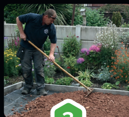
3 Lay the sub-base
