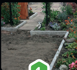
1 Remove soil and compact
